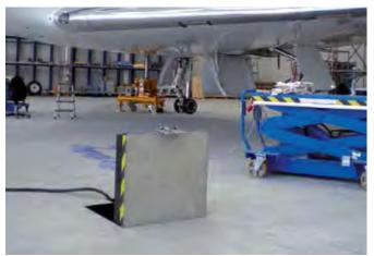
The GIFAS underfloor distributor PIAZZA 2000 has been specially designed for use at maintenance bases and in hangars.
