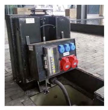
Solid stainless steel construction (V2A/1.4301) 580x580mm, load capacity up to 400kN, gas springs for fully automatic opening, shaft cover can be custom-filled, distributor as per the client's request.
